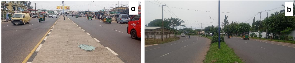
Figure 5. Comparison of contrasting pavement types at selected urban locations in Ilorin: (a) a recently constructed concrete surface that restricts direct stormwater infiltration; and (b) an unpaved vegetated surface that permits greater opportunities for infiltration. The comparison illustrates differences in surface permeability rather than measured runoff performance. Source: Author's field photographs, [August, 2025].
