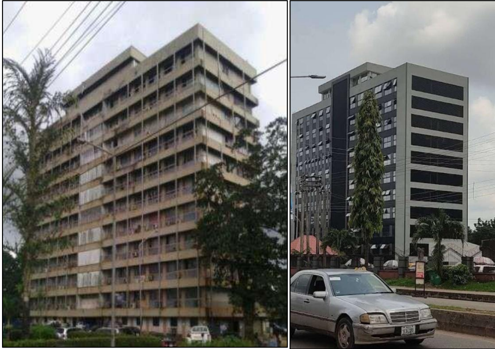
Figure 2 (a) Palm House before renovations. (Source: Research Gate / Okiemute et. al 2018)
