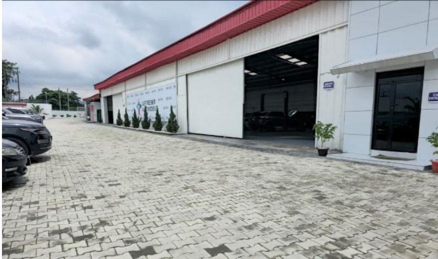
Figure 5. Workshop Facade with Sliding Doors and Roof Skylight for Combined Daylighting and Ventilation
