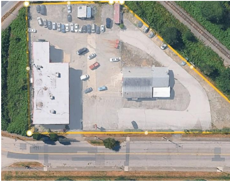
Figure 3. Site plan showing orientation and zone separation of spaces in an automobile training centre (not to scale).
