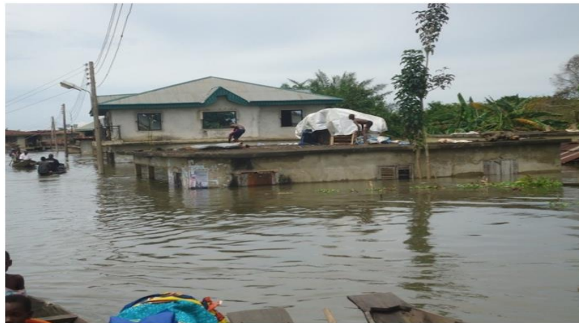
Source: (Ahmed Shittu THISDAY News Journal, May 28, 2017): Image of 2017 flooding at the downstream axis of Asa River: the area is one of the most affected by seasonal flooding
