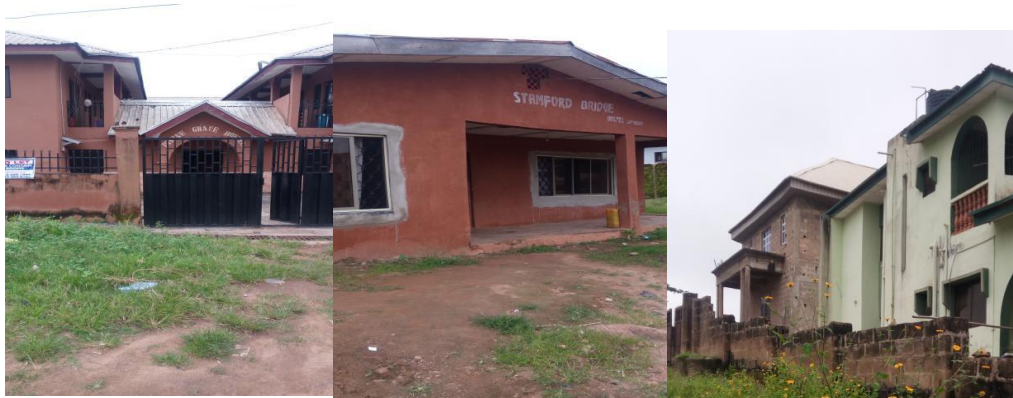
Plate 2: Student hostels constitutes about 60% of the buildings
